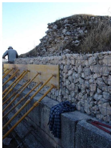
Figure 5: Structural consolidation. Clunia, Spain
